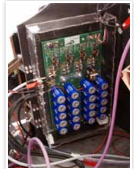
The boost converter causing most trouble this year.
